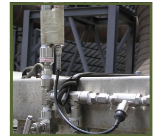
Orifice Plate Monitoring
